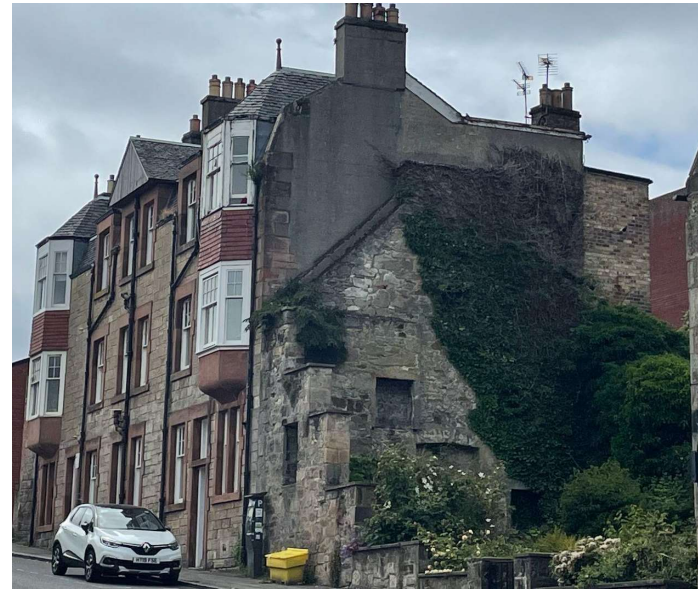
Station Masters House.
